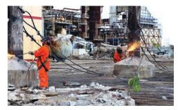
Structural steel towers, columns and structures were removed utilizing Brandenburg's specialized felling procedure. Once the razing of the structures were completed, hydraulic excavators with a shear attachment was used for process and recycling of the material. Brandenburg also utilized controlled explosives to demolish the 350-foot concrete stack.
